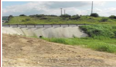
US 281 Concrete Rip-Rap Slope
